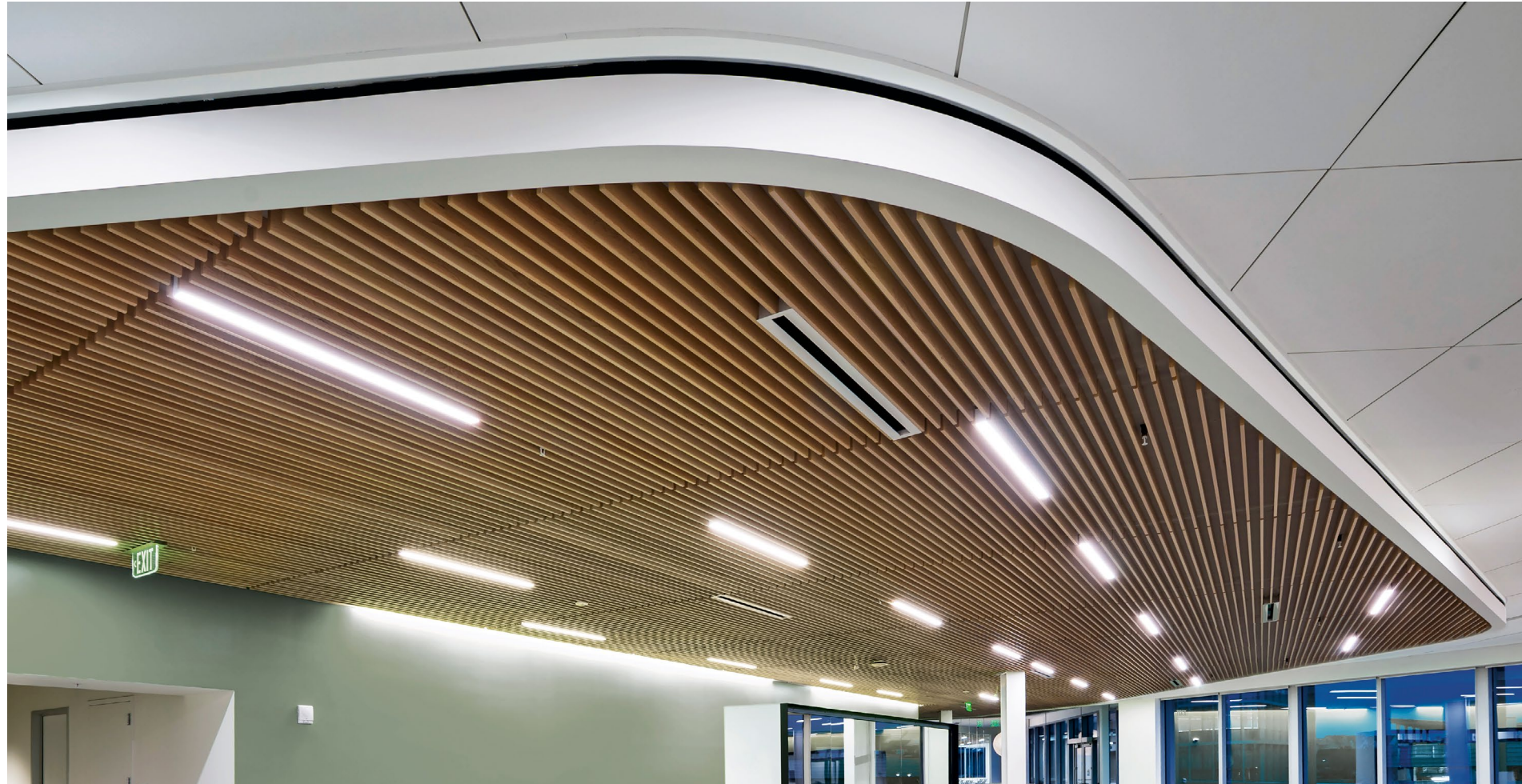
Armstrong® WoodWorks® Grille-Select Western Hemlock in a custom stain
