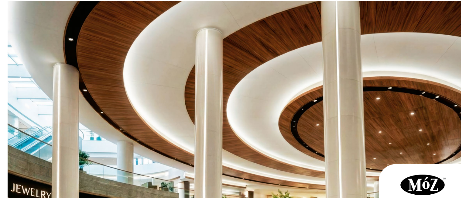
Móz™ Designs Luminous Columns with vertical Reveal Lighting
