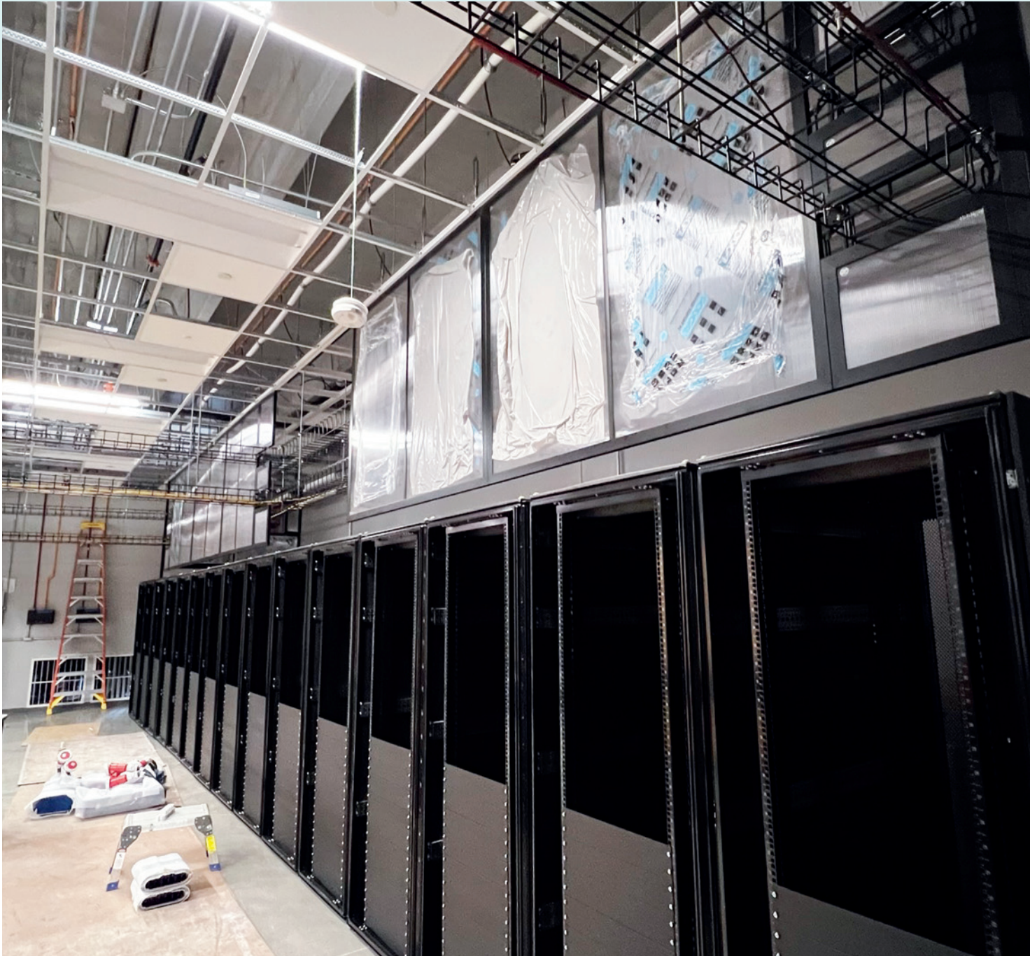
▲ DynaMax® Structural Grid with integrated air containment system from Subzero Engineering
