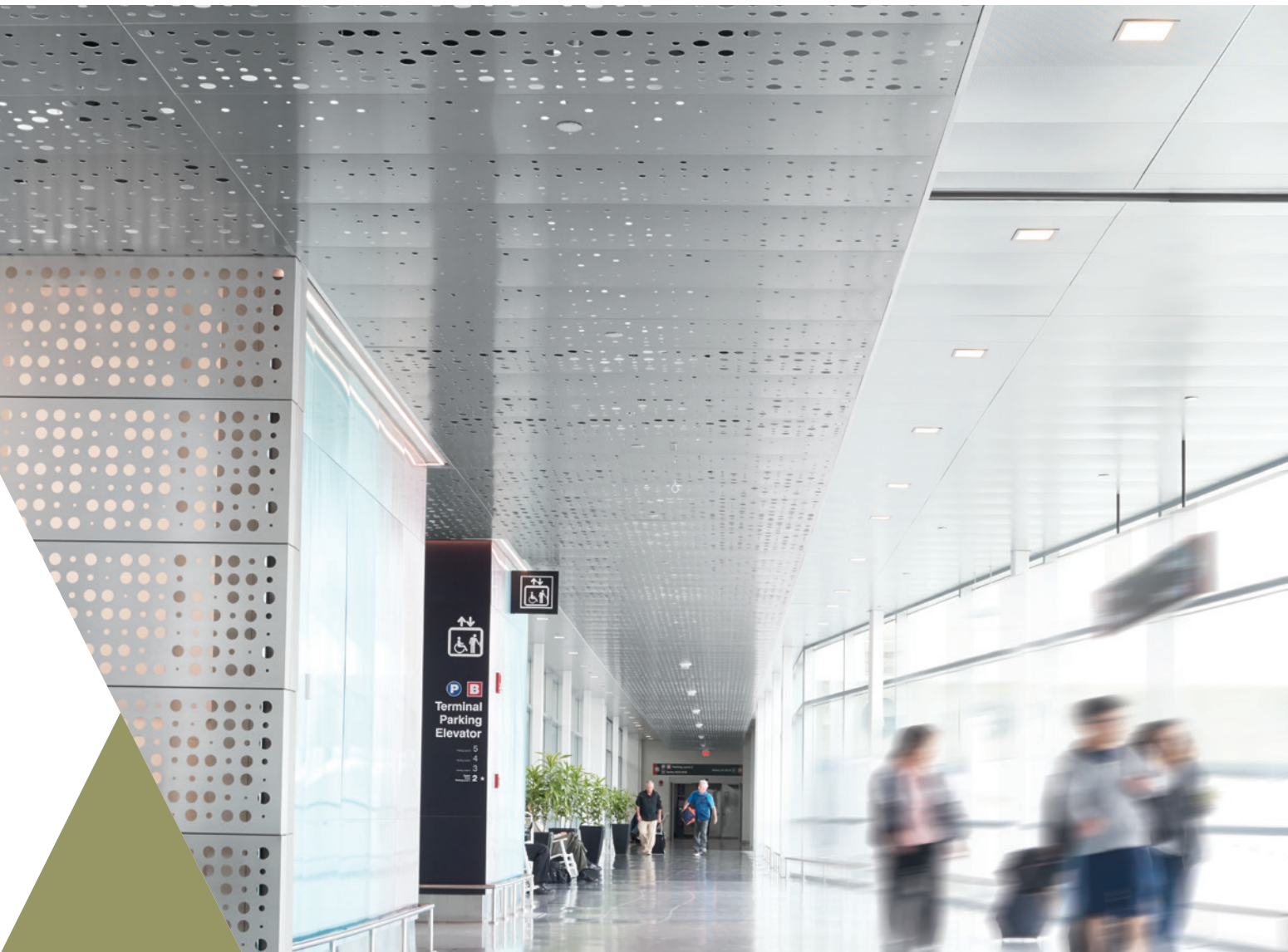
▲ MetalWorks™ RH200; Logan International Airport; Boston, MA; Arrowstreet, Inc., Boston, MA
