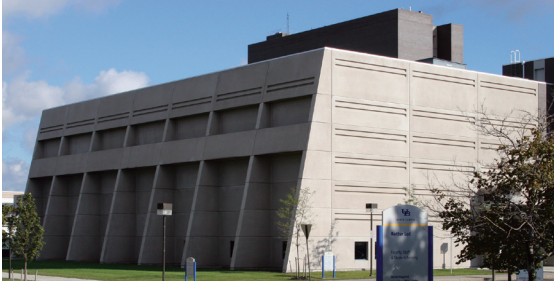
Exterior photo of UB's Structural Engineering and Earthquake Simulation Laboratory (SEESL)
