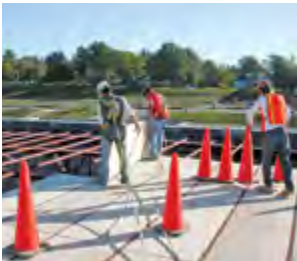
Tectum I Plank LWIC Installation
