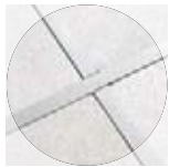
Ultima®/Optima® Square Lay-in with Prelude® 15/16"
