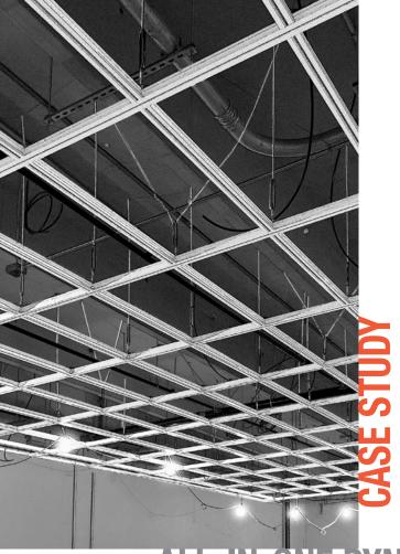
SITUATION Construct a structural data center ceiling to hang cable trays and equipment that also efficiently supports temperature and air containment systems
