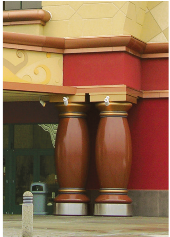
▲ Plasterform™ GFRC columns and cornices, and FRP signage and scrolls; Star Theatres, Various U.S. locations; FTC&H
