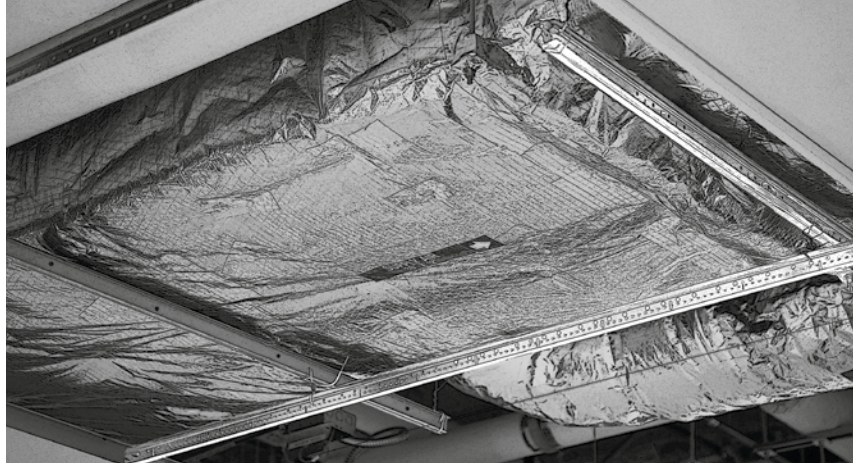
Trapeze Load Support with two main beams nested
