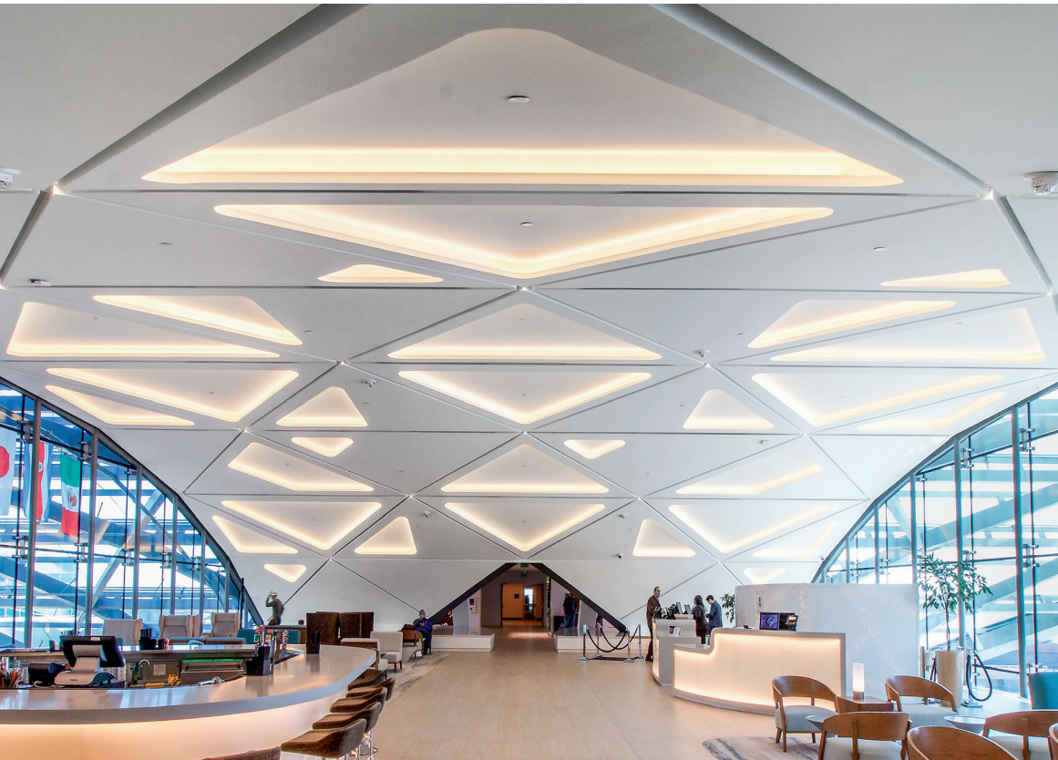
CastWorks GRG custom ceiling and wall panels with integrated light covers
