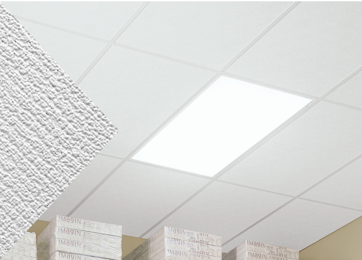
Shasta panel with Prelude® XL® 15/16" suspension system
