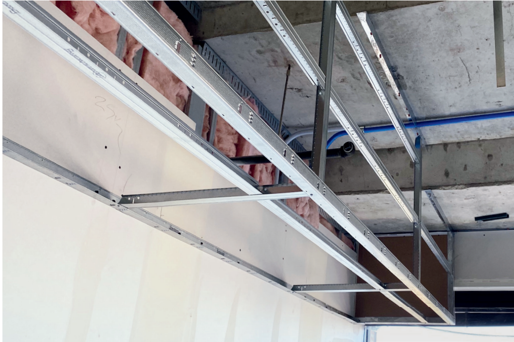
SimpleSoffit drywall soffit framing system, part of the FrameAll™ Drywall Grid family of products
