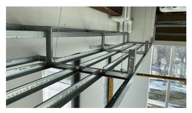
LANCASTER, Pa. — Armstrong Ceiling & Wall Solutions has introduced the SimpleSoffit™ Drywall Framing System, a new prefabricated grid solution that provides a faster, easier, better way to build drywall soffits in complex and labor-intensive configurations.
