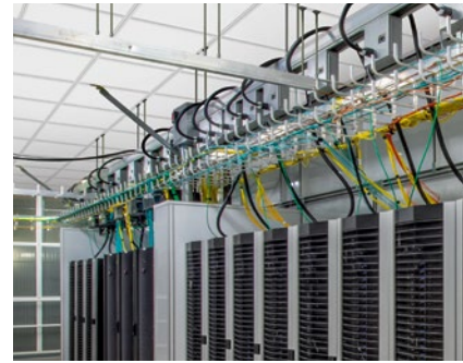
DynaMax Plus Structural Aluminum Suspension System
