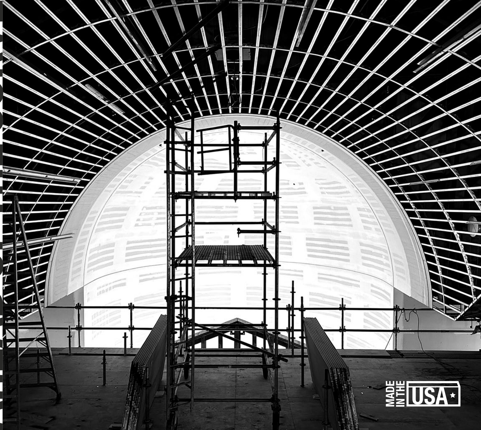
Flat Drywall Grid barrel vault installation
