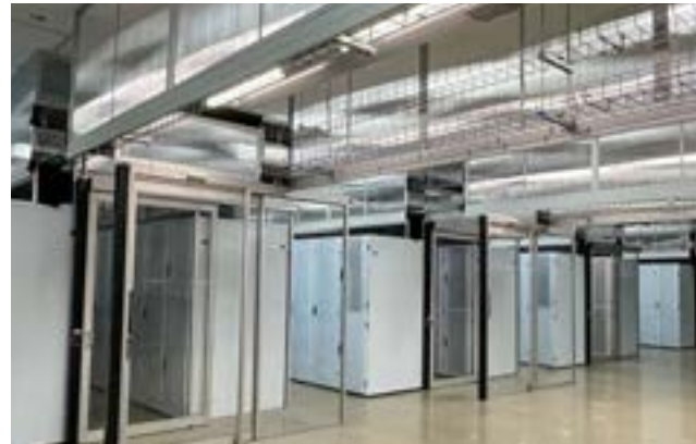
Ultima® AirAssure™ low leakage ceiling panels and DynaMax® structural grid.
