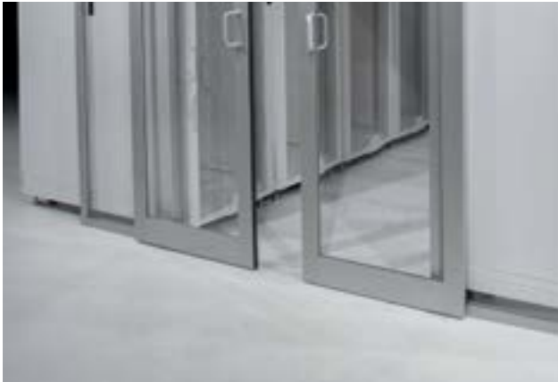
Slab Floor Data Center
