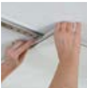
3 Position tile or plank; slide and secure clip
