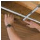
Position planks; slide and secure clips
