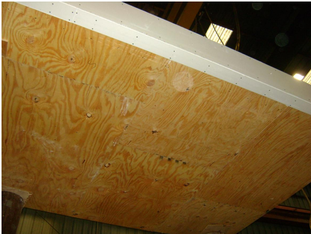
Figure 5. Exposed surface of prescriptive code compliant floor/ceiling assembly.
