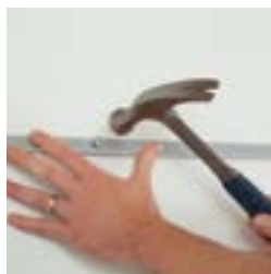
1 Install wall molding
