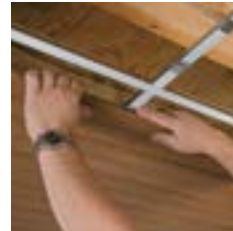
Position planks; slide and secure clips
