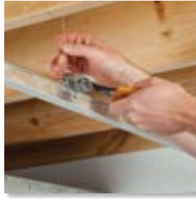
2 Suspend main beams with hanging hardware
