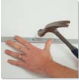
1 Install wall moldings
