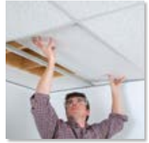
4 Install ceiling panels
