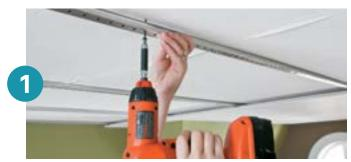
Attach metal tracks (item #1190) perpendicular to ceiling joists
