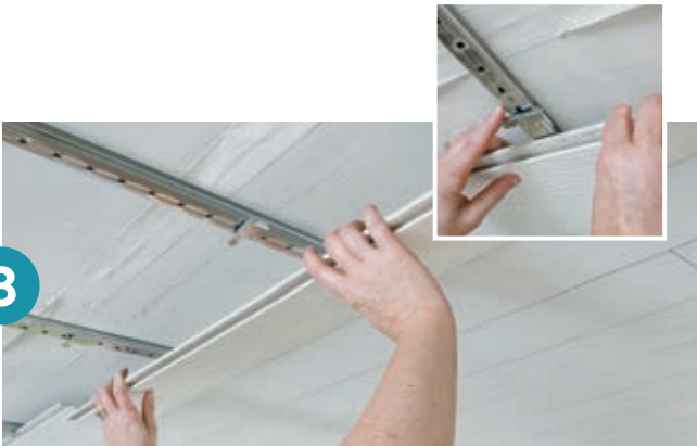
Position tiles or planks; slide and secure clip
