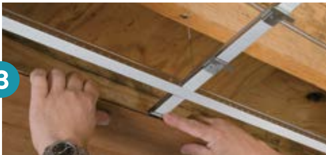
3 Position planks; slide and secure clips
