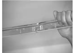
Join sections of main beam
