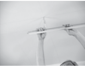
Install first main beam
