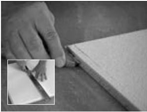
Tegular-edge border panels may require field cutting. Cut border panels face up and paint edges
