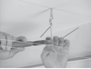
Bend hanger wires at height of guide string
